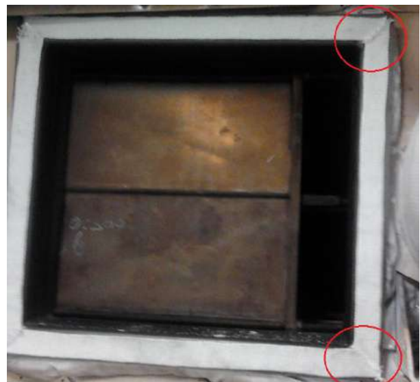
Image x Example of positioning of the gasket on the hatch
